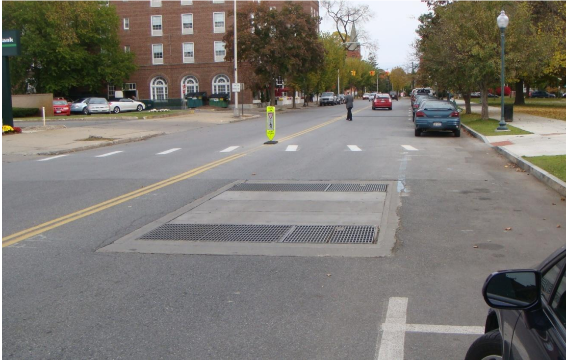
Photo 2. Position of grate in the street.
